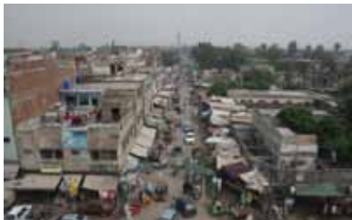
General view of the road condition
