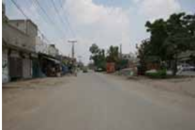
General view of the road condition
